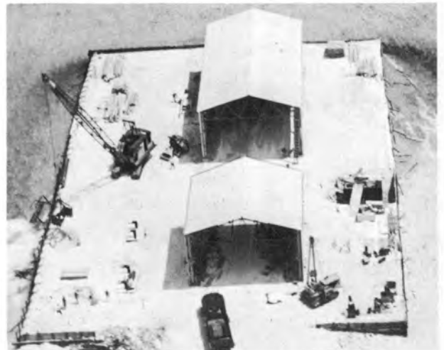
Figure 2-55. Stations 311.01 and 310.02 50% Complete - Man-Made Island No. 2
